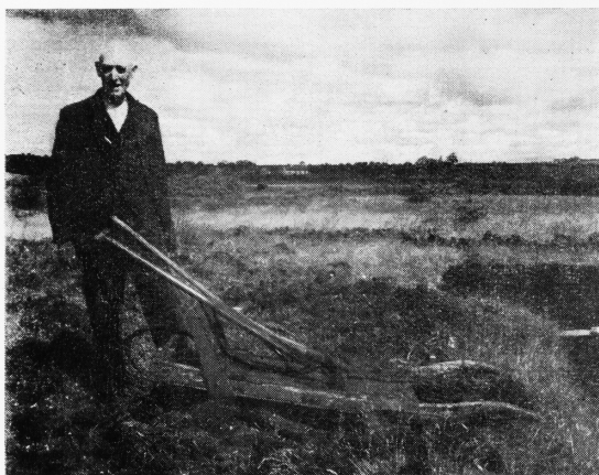
Plate VII. (a)—Left—D. Gordon, Bowbrig Farm, with his peat-cutting equipment in Drummoddie Moss. (b) Right—The dried-out top of D. Gordon's peat bank, showing the cuts made by the draining spade, and the mug tile in position on its sole. The softer peat starts immediately below the level of the tile.
