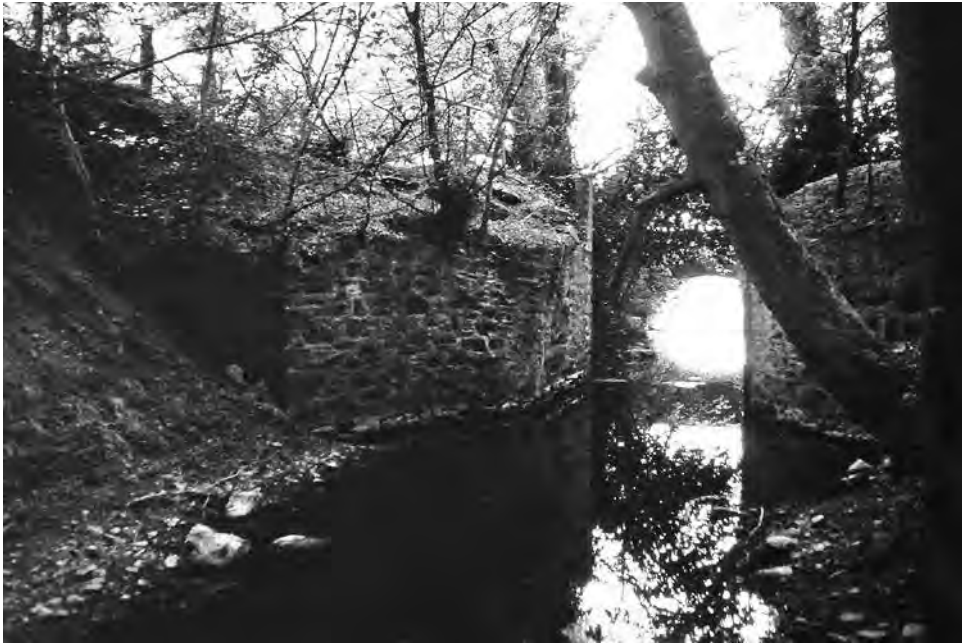
Figure 1. Buchan's bridges, viewed in the late 1970s; the abutments of the original bridge, the present bridge in the background, and some of the stone rubble dumped into the former canal to raise the level of Carlingwark Loch. (Photograph: John Howat)
