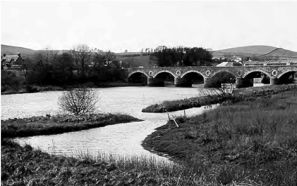
Figure 7. Glenlochar Bridge in the late 1970s. The Culvinnan Canal's partially filled entrance from the river Dee shown on Ainslie's 1797 map, and its c. 1801 northern extension's pile-protected banks, viewed from the embankment shown on early OS maps (Figure 5). (Photograph: John Howat)
