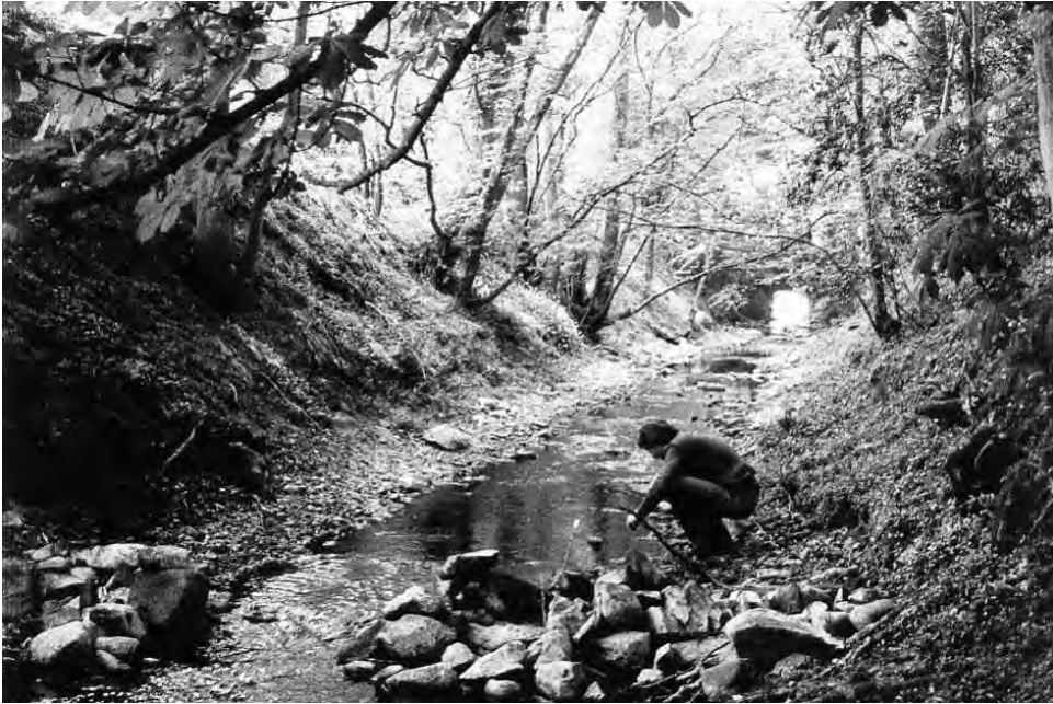
Figure 2. Buchan Cutting. The disused Carlingwark Canal in the late 1970s, long since reduced here to a rubble-filled drainage channel or 'Lane', looking up the cutting towards Buchan Bridge from beside Carlingwark House. (Photograph: John Howat)
