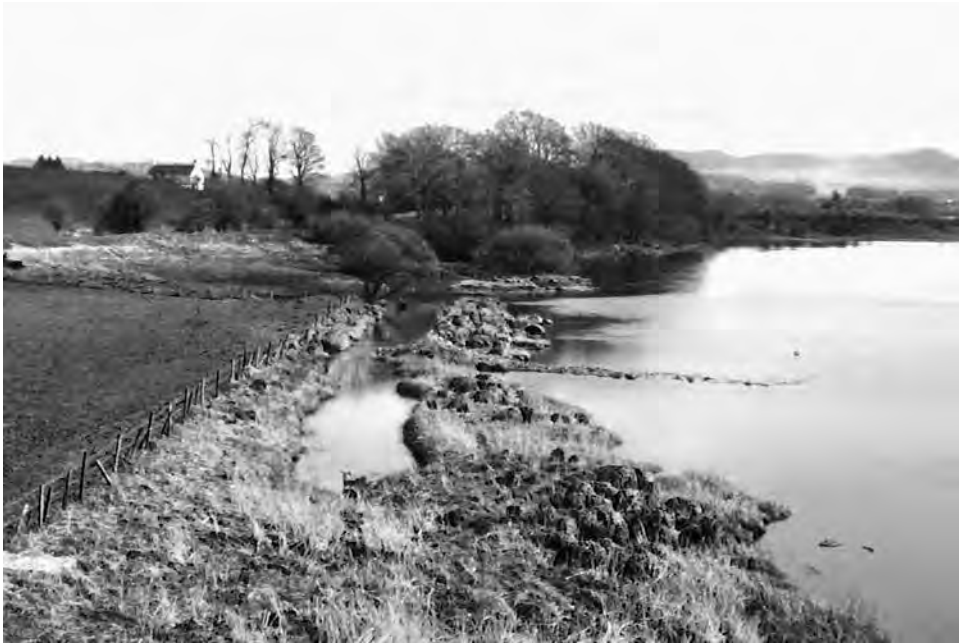
Figure 6. The northern extension of Culvennan Canal beside Abbey Field (or Abbey Yard) viewed from Glenlochar Bridge in the late 1970s. Note what appear to be the remains of a stone-rubble weir; it would have needed to raise the river's surface by at least two feet in summer low-flow conditions, but a weir did not exist in 1802. (Photograph: John Howat)
