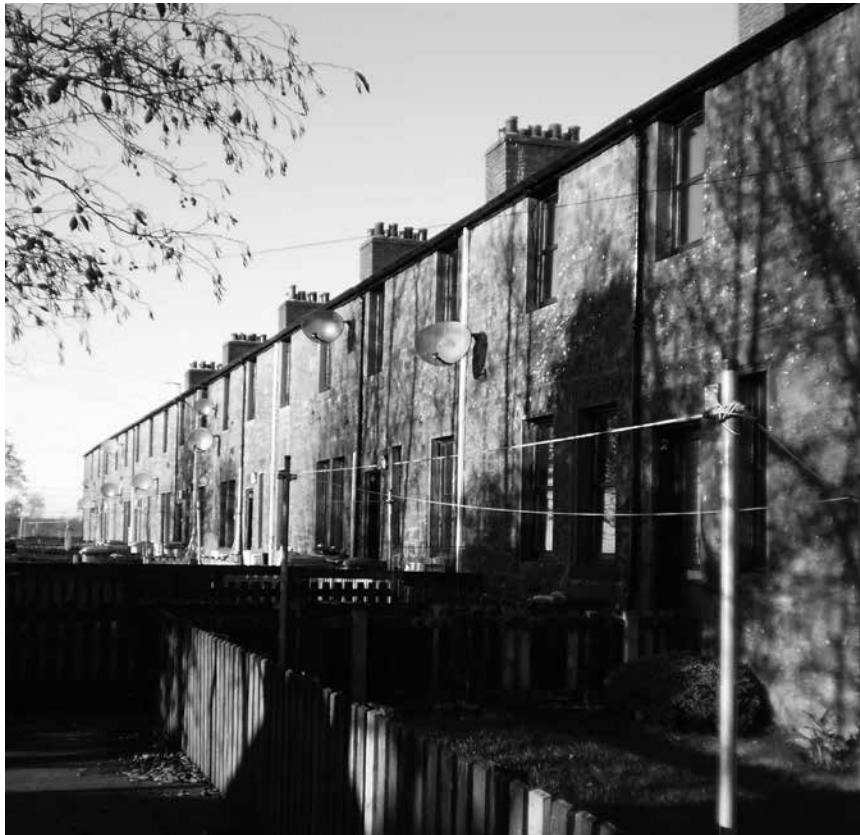
Figure 6. The back of Victoria Terrace in 2013: satellite dishes where in the 1930s these were the outdoor toilets, wash houses, and middens.
