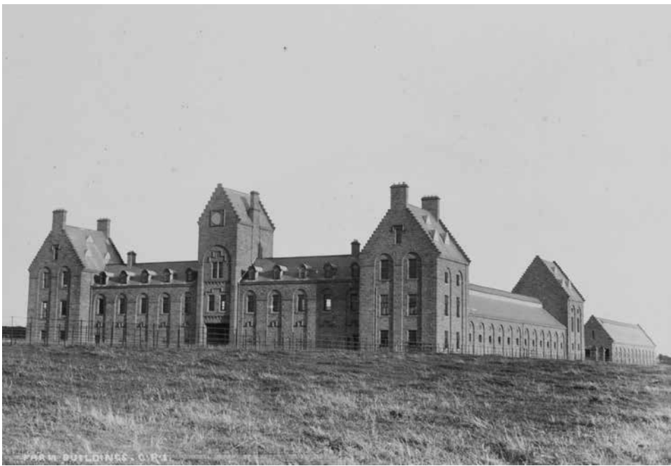
Figure 28. Farm buildings, north (left) and west (right) façades. (Album 4, number 28)
