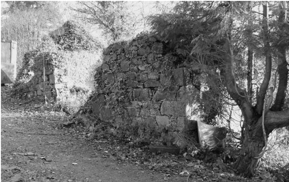
Figure 9. The west wall from the south-west.
