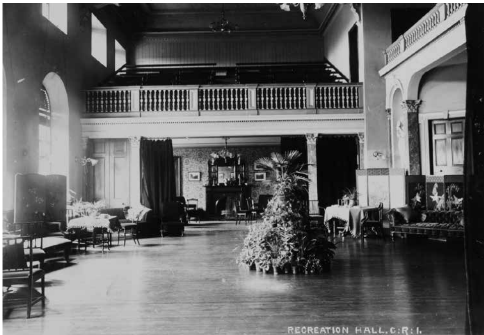
Figure 18. The Recreation Hall. In the 1890s there were three balconies. The one on the right still exists. (Album 4, number 16)
