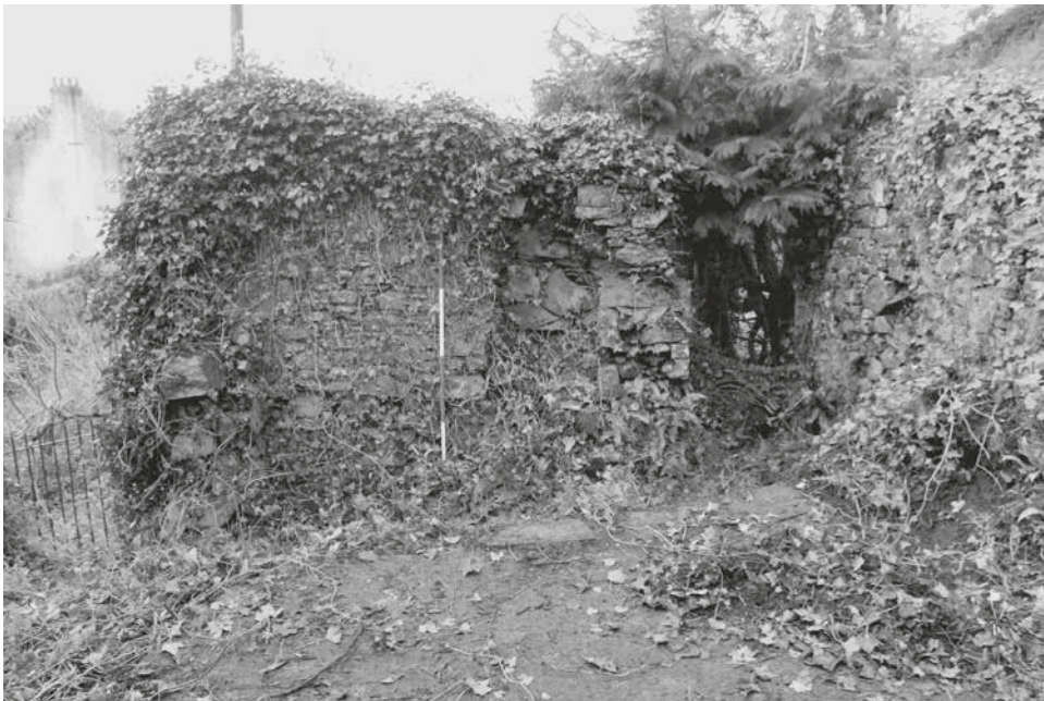
Figure 8. Internal view of the south wall. Note fireplace to right of range rod and door in south-west corner.
