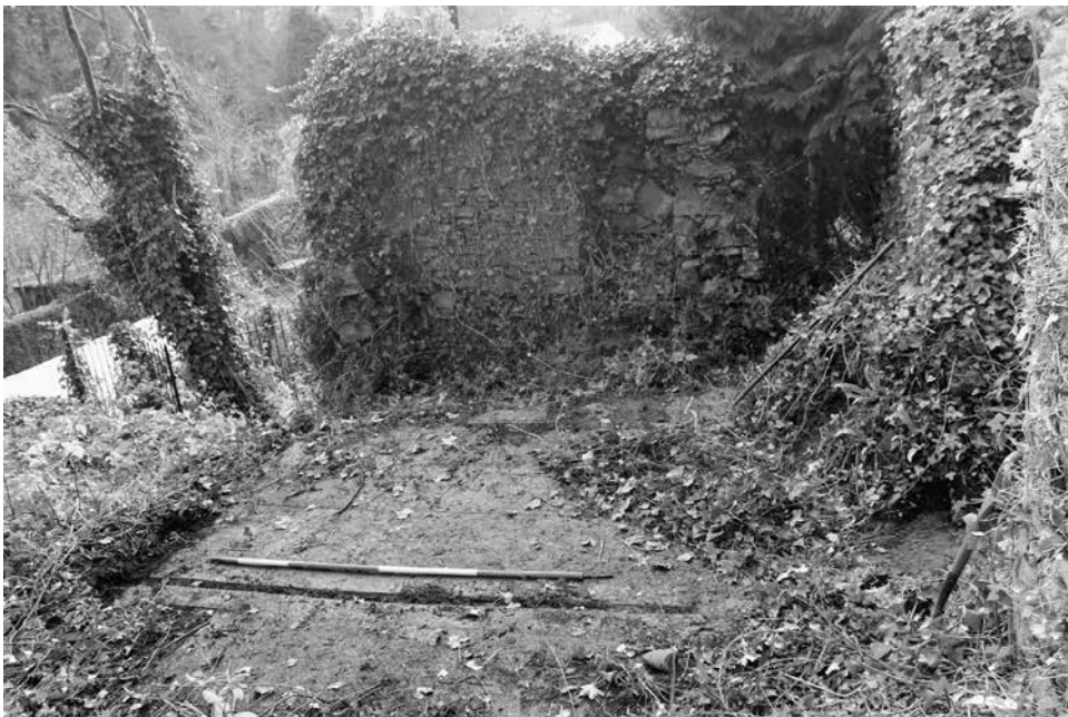
Figure 4. The concrete floor (floor 27) and drainage channel, from the north.
