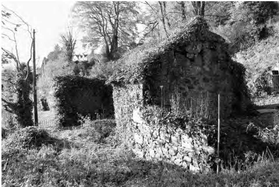
Figure 3. The north extension (walls 9 & 10) from the north gable.
