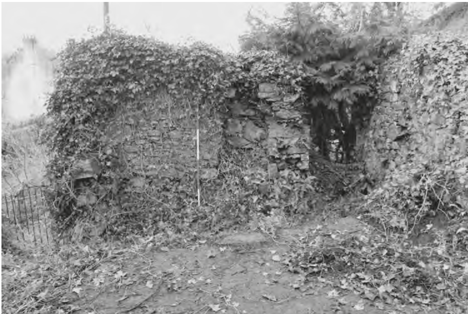
Figure 8. Internal view of the south wall. Note fireplace to right of range rod and door in south-west corner.
