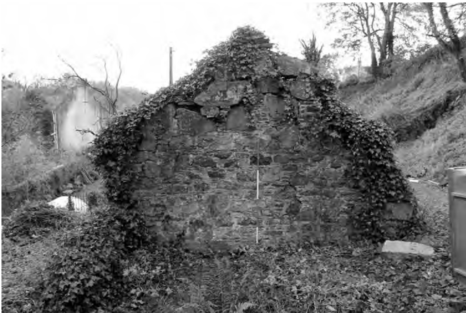
Figure 10. The extension (walls 9 & 10) and north gable wall (wall 7) from the north.
