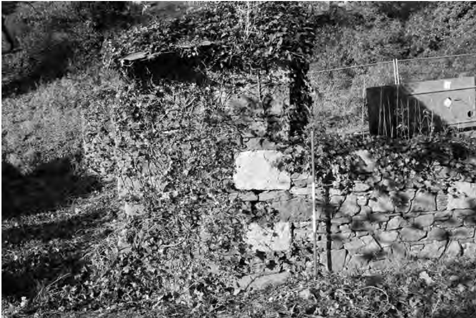
Figure 11. North end of the east wall (wall 11) with roof slates on the wall head, from the east.
