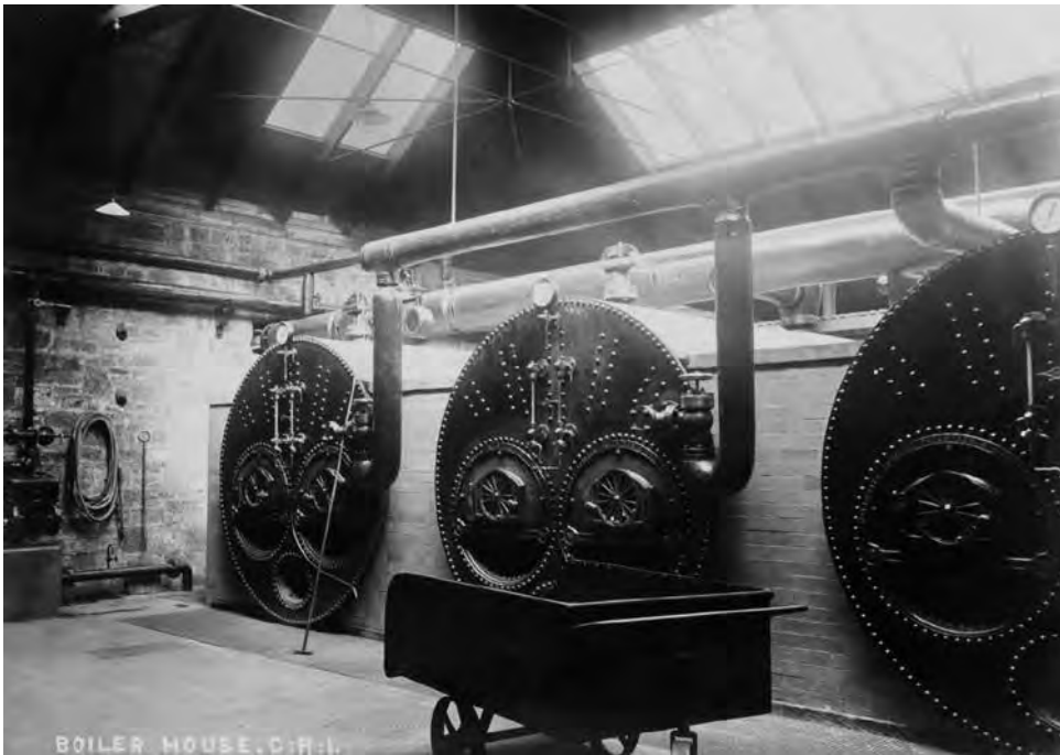
Figure 34. Boiler house. (Album 4, number 37)
