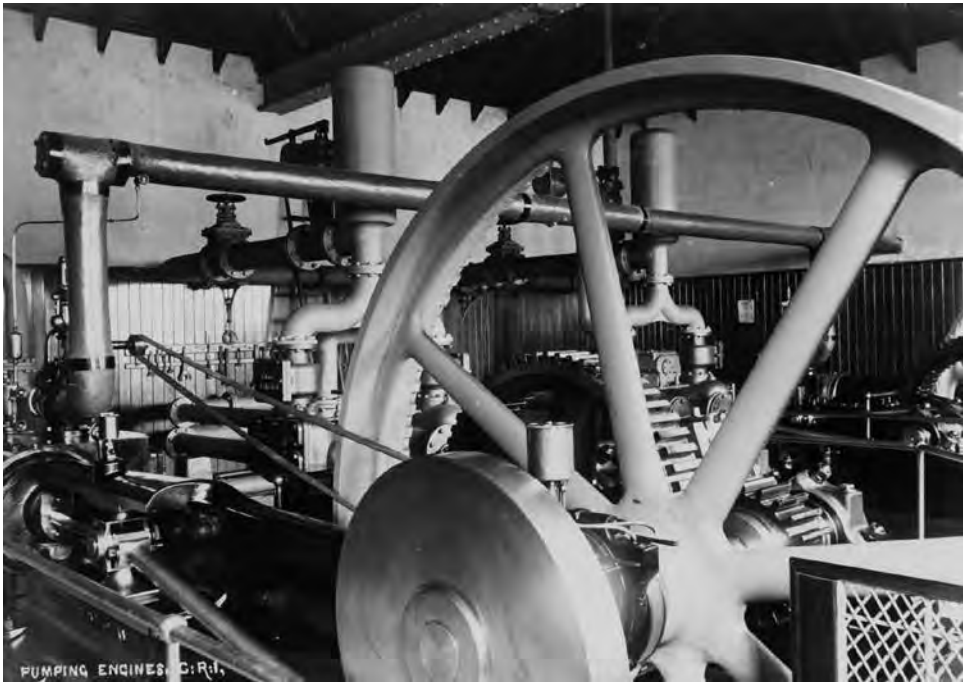
Figure 37. Pumping engines at the artesian well. (Album 4, number 42)
