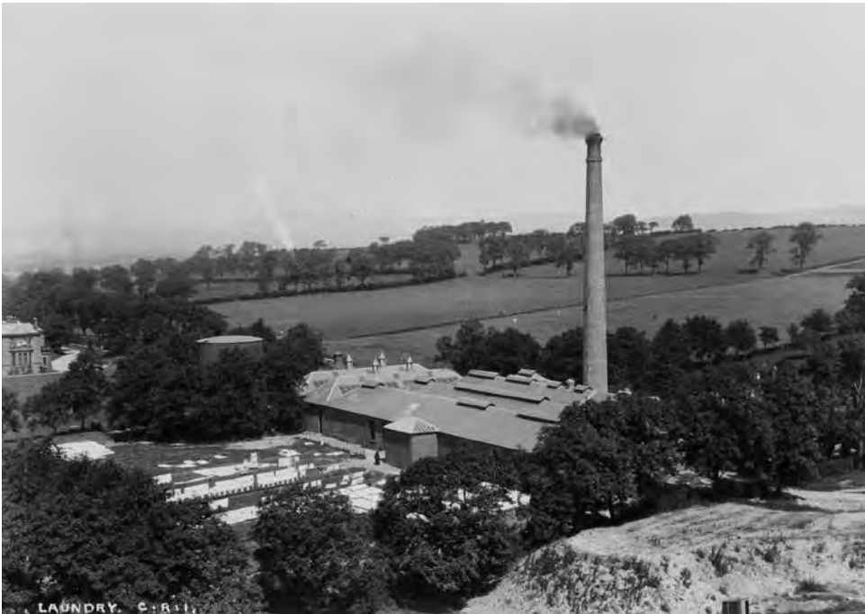
Figure 23. Laundry, taken from the newly erected church tower and showing the laundered items literally on the 'drying green'. On the extreme left in the Physician Superintendent's house and on the right is the former water tower. (Album 4, number 23)
