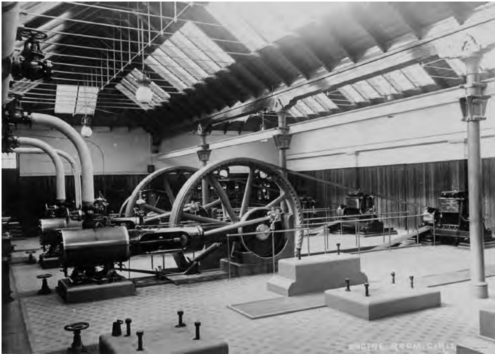
Figure 31. Engine room of the electricity generating station. (Album 4, number 34)
