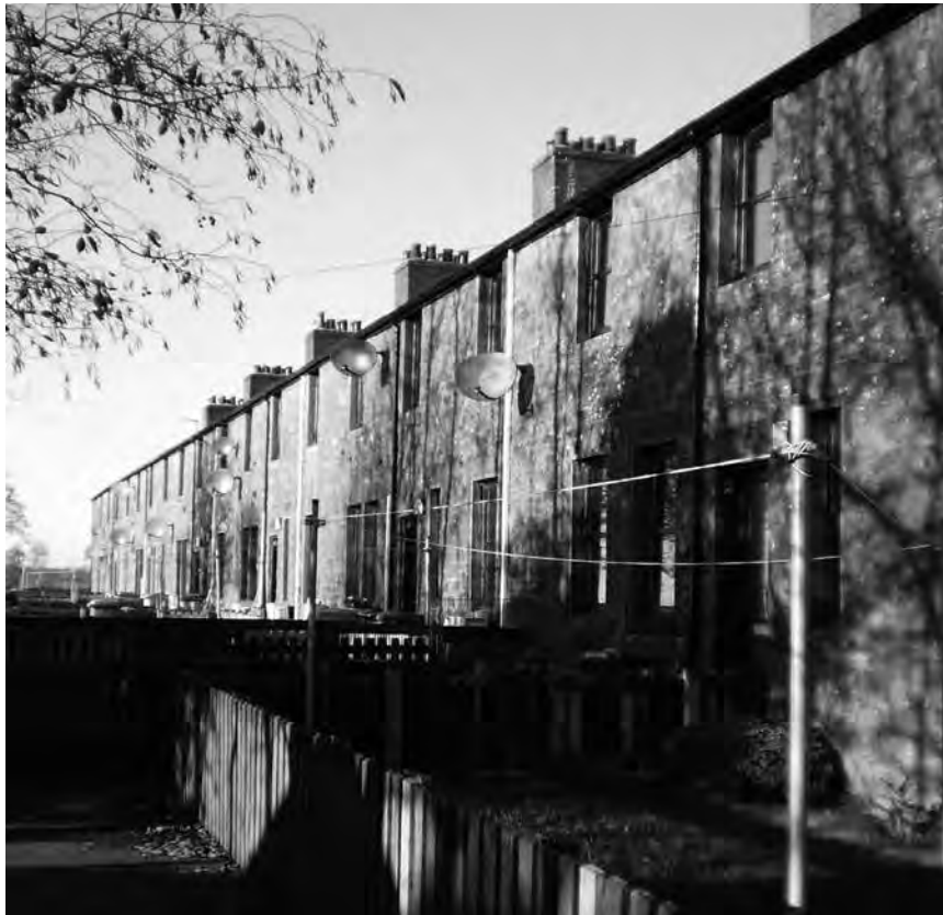
Figure 6. The back of Victoria Terrace in 2013: satellite dishes where in the 1930s these were the outdoor toilets, wash houses, and middens.
