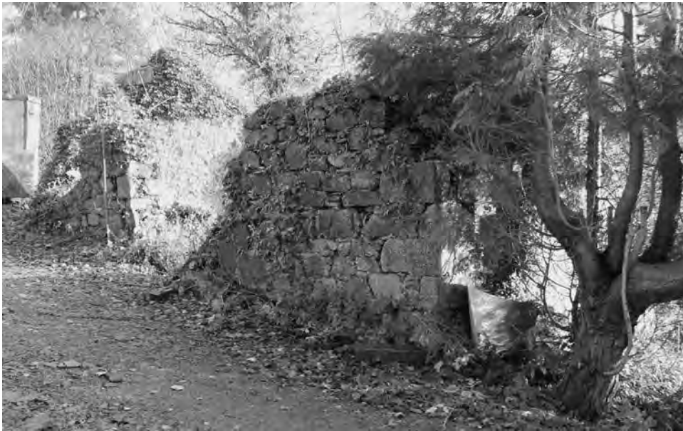
Figure 9. The west wall from the south-west.
