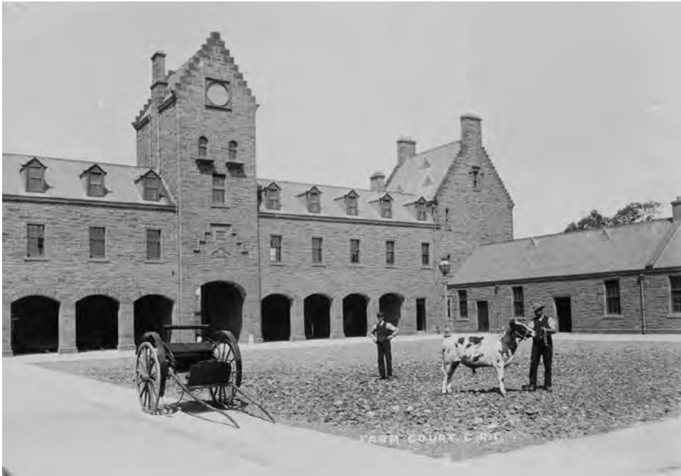
Figure 27. Farm court. The central archway was built up and other arched areas were glazed in the early twentieth century. (Album 4, number 26)
