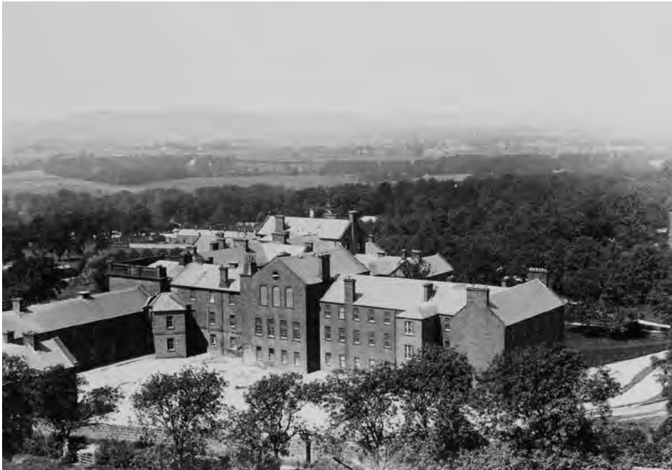
Figure 26. Rear of Second House. It was demolished in stages in the first quarter of the twentieth century. (Album 4, number 25)
